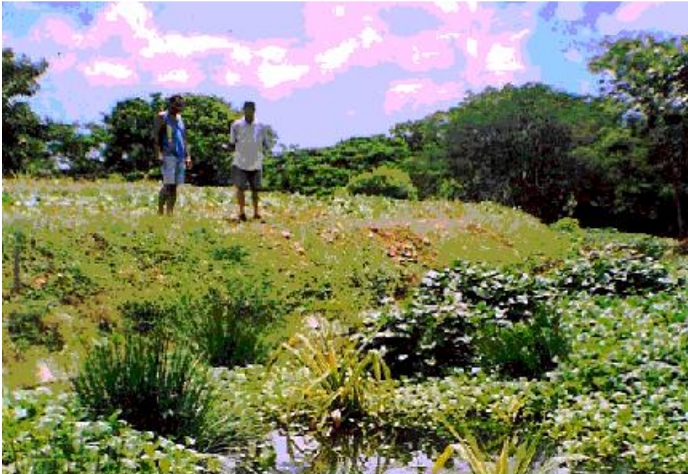
Completed wetland planted with a variety of species
